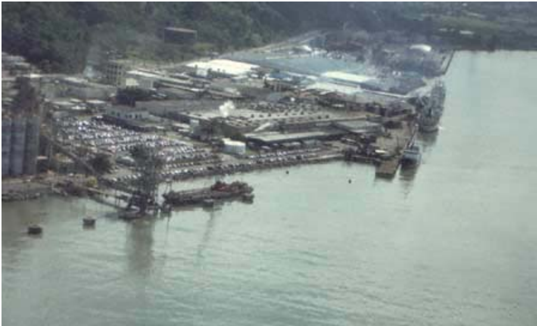
Figure 12. Mayagüez harbor, docks and seawall
