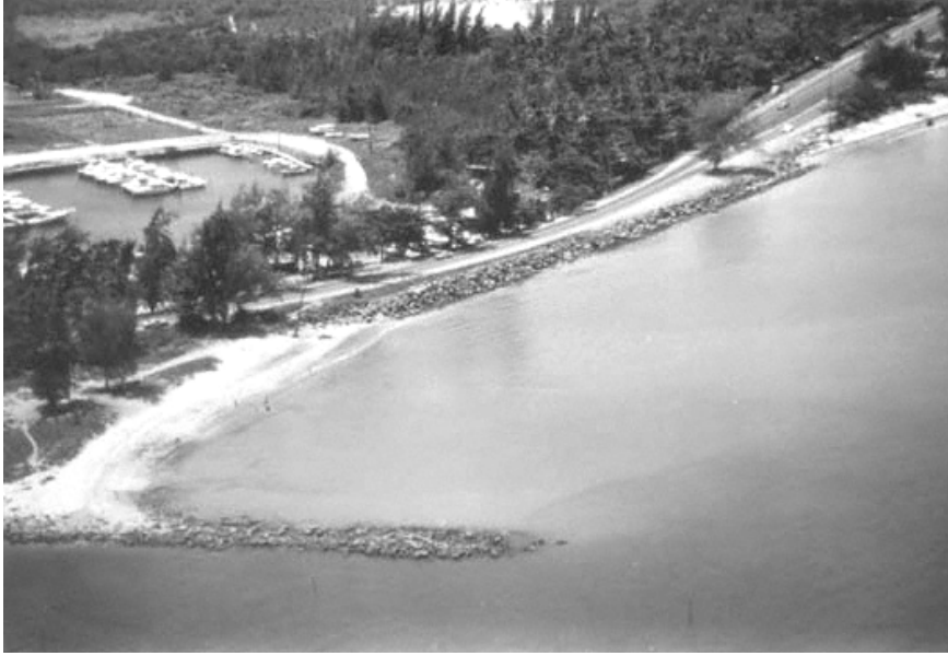
Figure 11. Boca de Cangregos jetty and riprap
