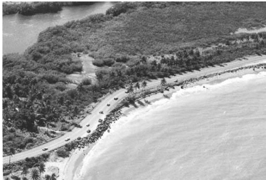
Riprap of boulders
