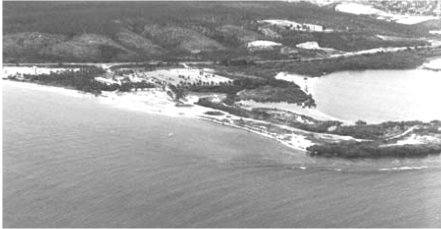
Figure 15. Erosion, groyne and breakwater at El Tuque
